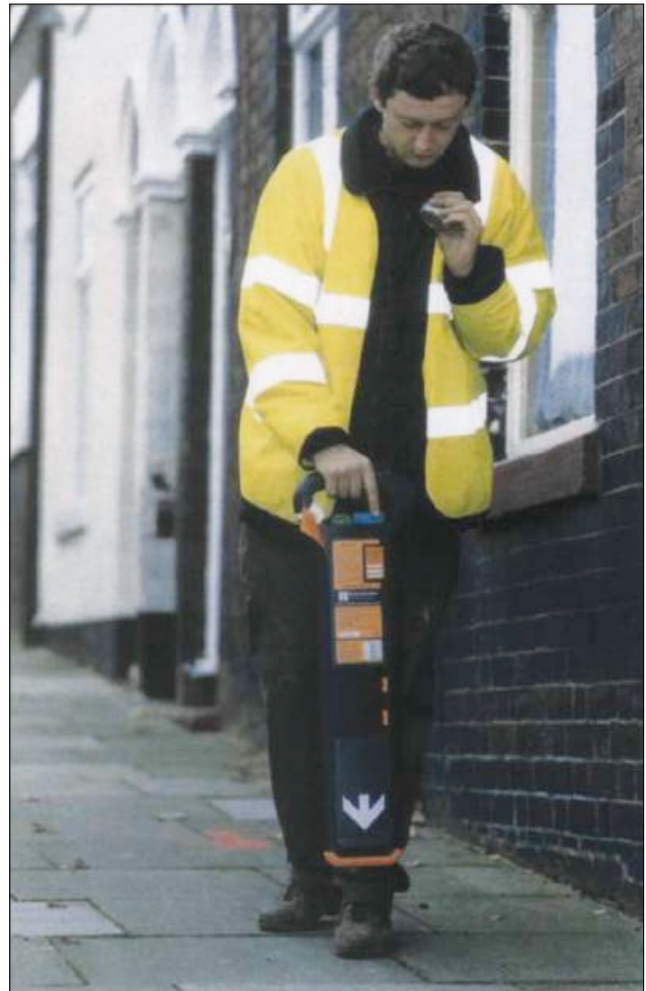
Figure 5 Using a cable locator
