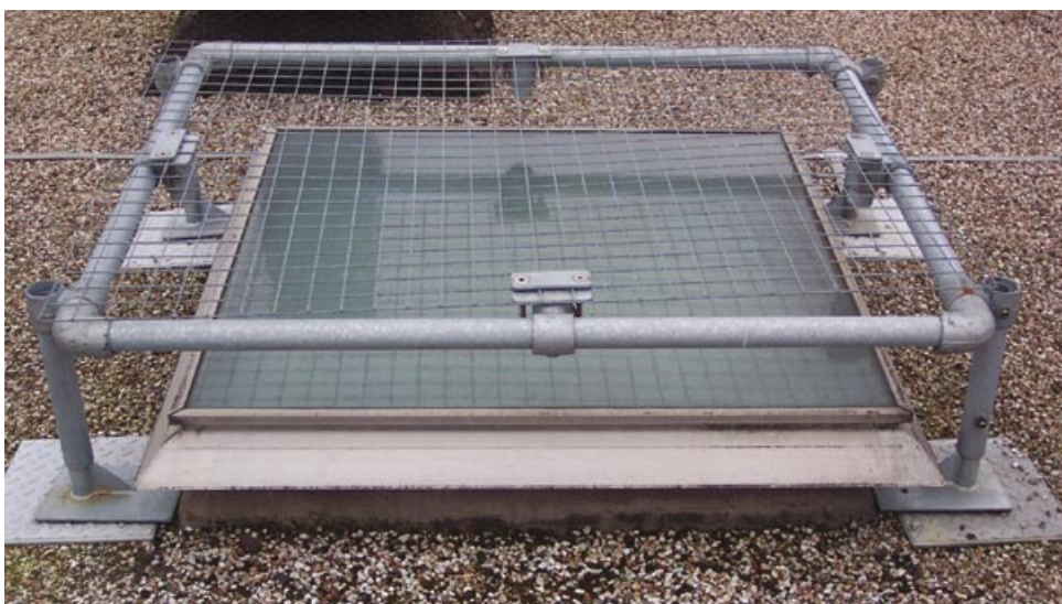
Covers can be fitted to existing roofs or included as part of the design (Image courtesy of Safesite)
