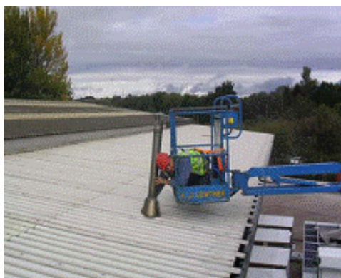
Using a MEWP to inspect a vent
