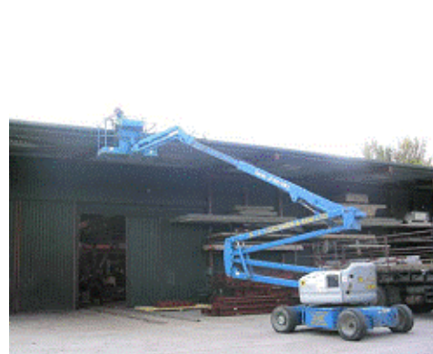
Using a MEWP to clean a gutter
