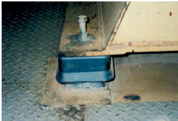
Figure 7 Detail of vibration-isolating mount
